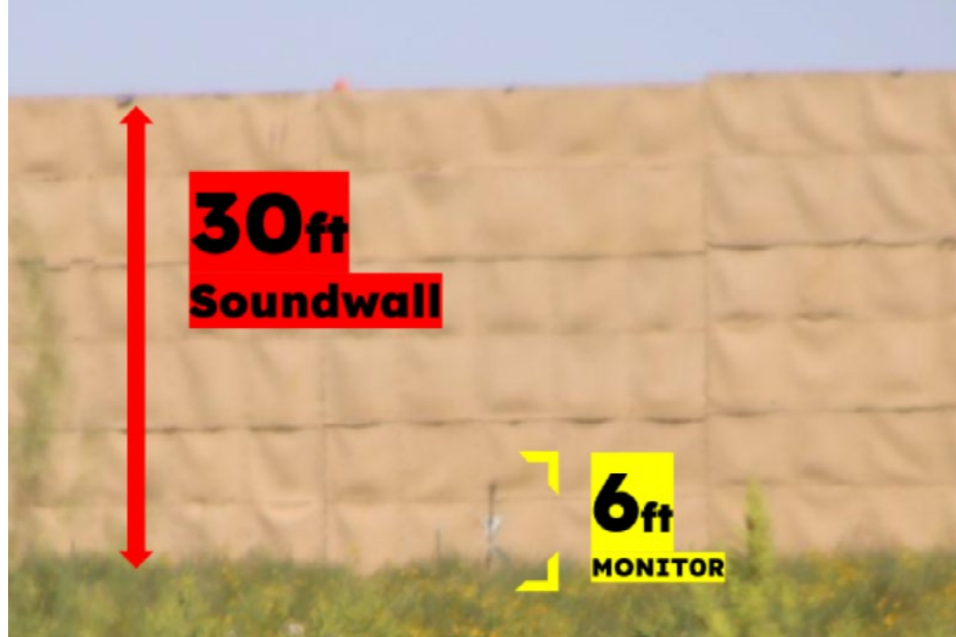
Image illustrating size and placement of a monitor in relation to a soundwall surrounding an O&G site in Colorado.
